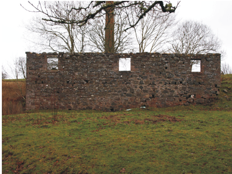
Illus 6 Mill House 02, N Elevation. Chimney 01 behind.
