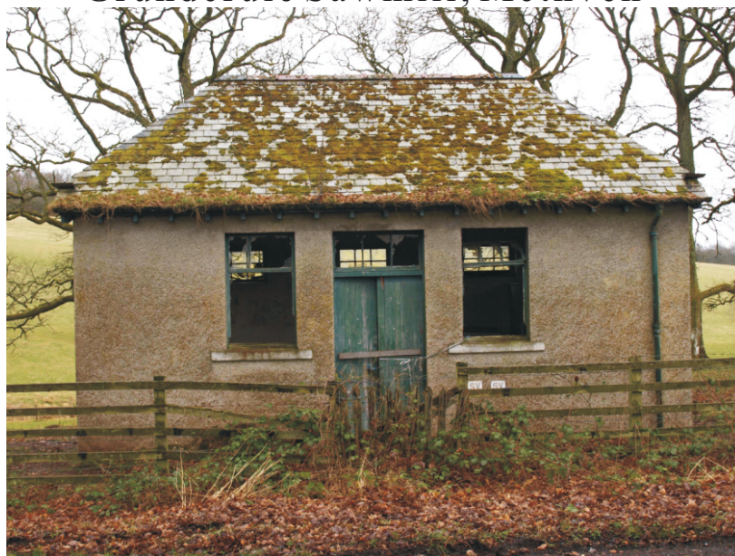
Illus 12 Water Treatment House 34 from road.
