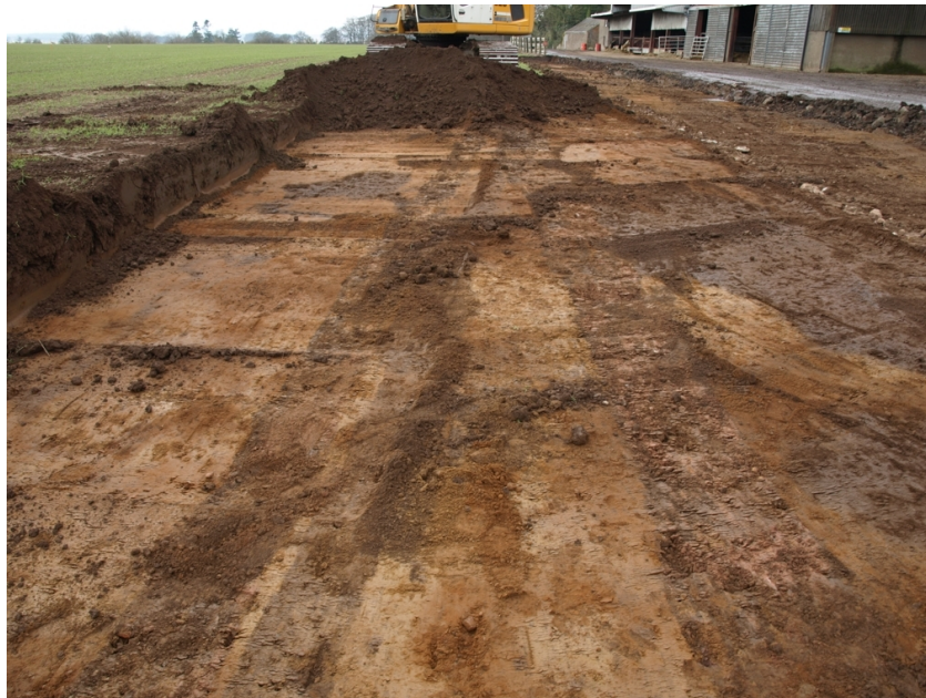
Field drain and water pipe trenches in natural sand, looking W
