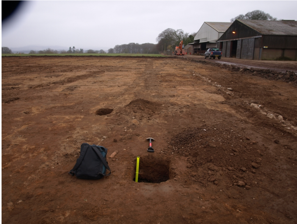
Illustration 4: Sondages in water pipe trench 05 and field drain trench 03, looking W.
