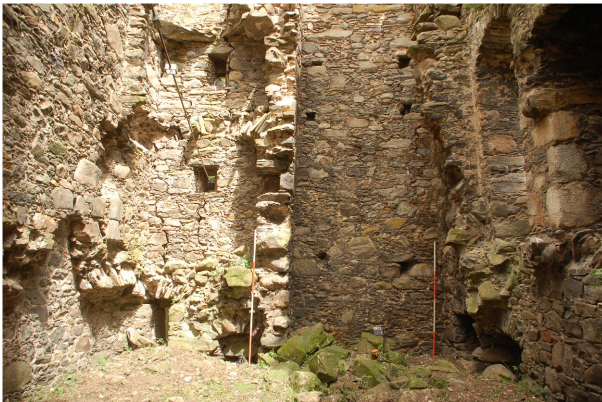
Image 6: Base of N elevation, interior of main building, with “oratory” to left of flue
