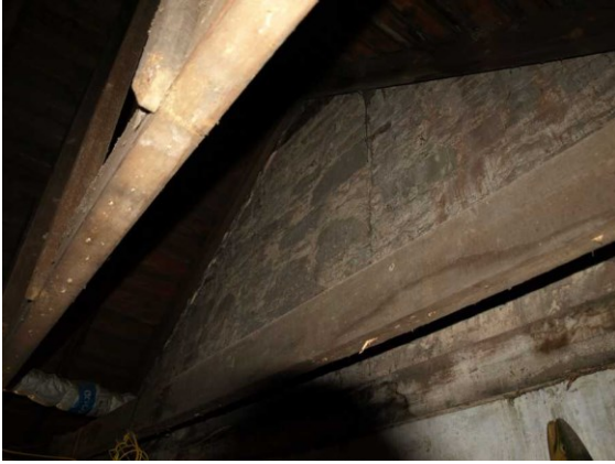
Illustration 18: W Range Loft. Blocked opening in E wall?
