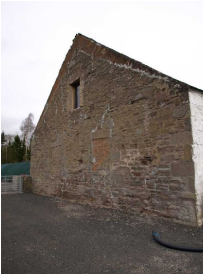
Illustration 7: W gable. Blocked openings, inserted window and raised roof line
