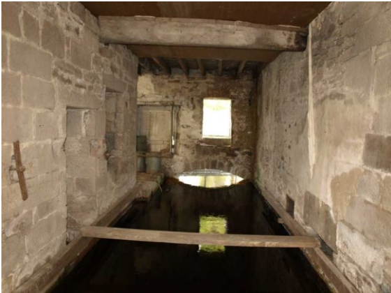
Illustration 13: Internal mill lade, N. Wheel mark on wall
