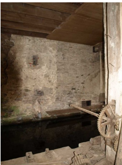
Illustration 14: Sluice mechanism in W Range
