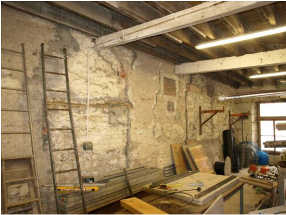
Illustration 12: W gable of W Range. Blocked openings, and floor timbers above
