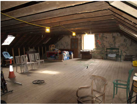
Illustration 16: W Range Loft. Inserted window in W gable
