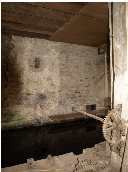
Illustration 14: Sluice mechanism in W Range
