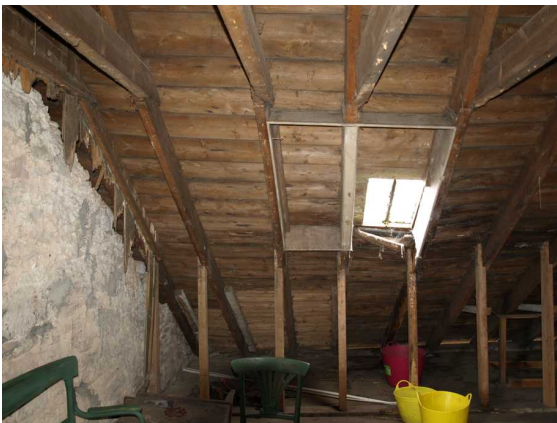
Illustration 17: Reduced roof light in NW corner. Traces of lining boards on W gable wall.
