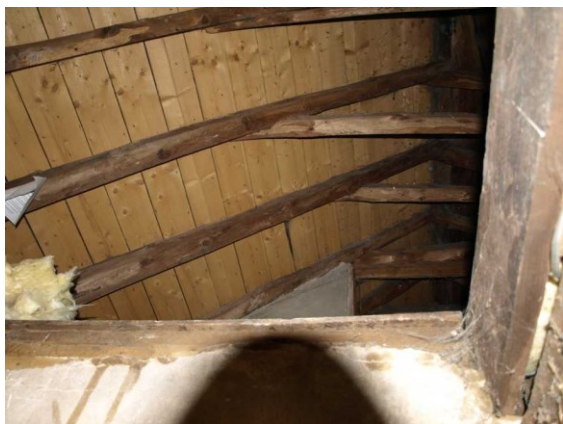
Illustration 27: The Farm House. Roof timbers in loft.
