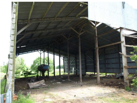
Illustration 20: The E Barn, internal structure.
