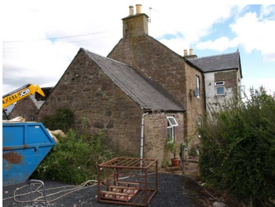
Illustration 21: The Farm House. W gable end and W extension.
