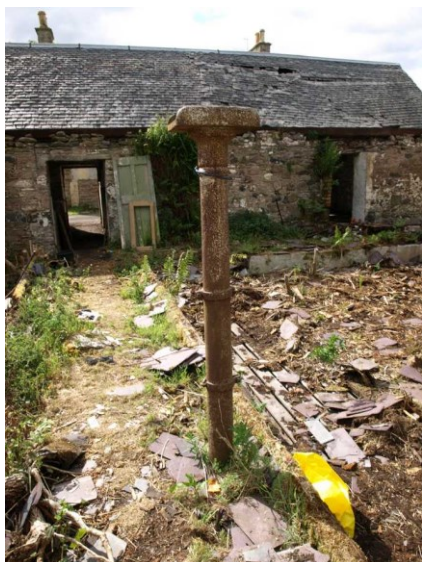
Illustration 12: Detail, cast iron column in Courtyard.
