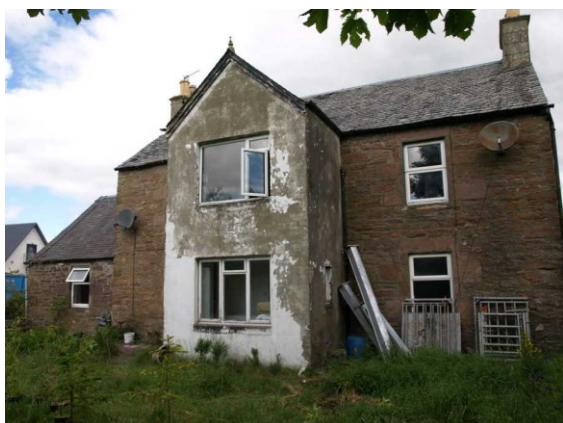
Illustration 22: The Farm House. S elevation and S extension.
