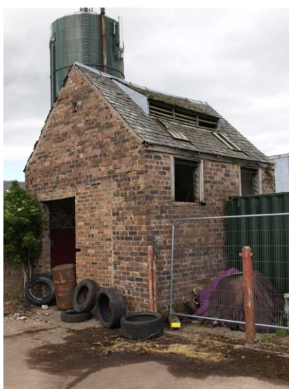
Illustration 17: The Dairy, S gable end with reduced doorway.
