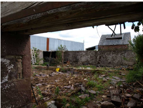
Illustration 11: The Courtyard. Ventilation slits in E wall.
