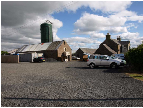
Illustration 6: General view, N. W Range, Farmhouse, Grain Silo and S Range beyond.
