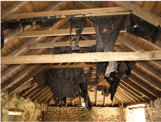
Illustration 16: S Range, interior. Roof timbers at E end.
