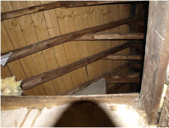
Illustration 27: The Farm House. Roof timbers in loft.
