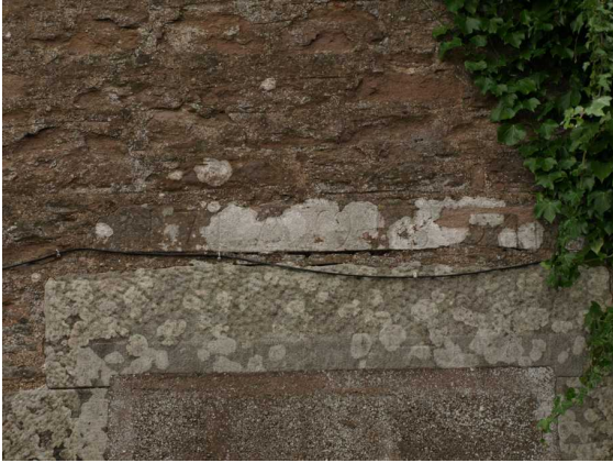
Illustration 9: W Range, detail of re-used marriage lintel.
