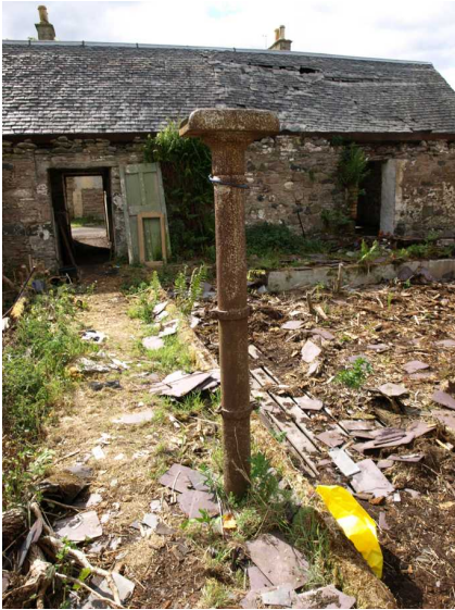
Illustration 12: Detail, cast iron column in Courtyard.
