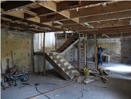
Illustration 24: The Farm House. Ground floor interior with central stair.
