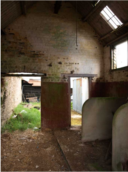
Illustration 18: The Dairy, interior. N gable end with double doorways. Stalls in E wall.
