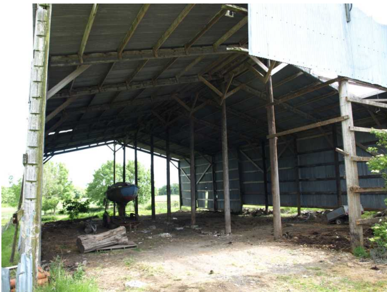
Illustration 20: The E Barn, internal structure.
