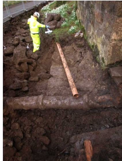
Illus 7 Foundation 014 and slab 020 under tower and buttress.
