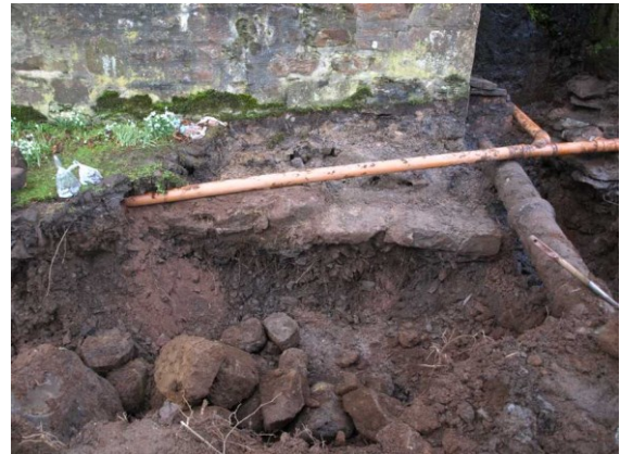
Illus 8 Foundation 014 and slab 020 under tower and buttress (R). Bedding 015 and rubble 012 under foundation 014.
