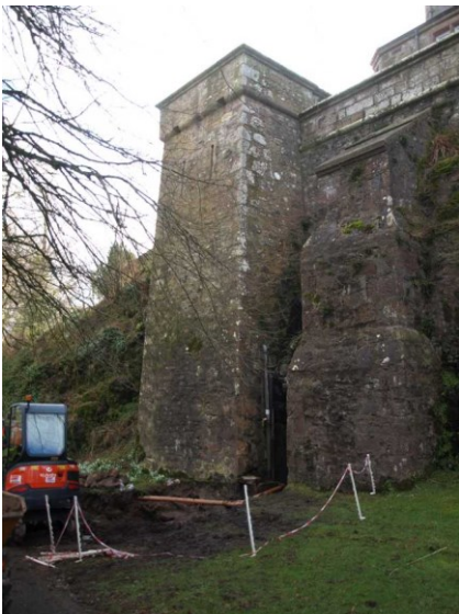
Illus 10 Tower and buttress on foundation 014 and slab 020.
