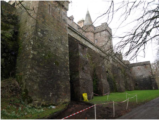
Illus 4 Tower and buttresses against cliff face.
