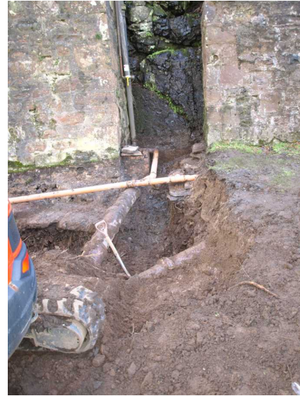
Illus 11 Foundation 014 and slab 020 under tower and buttress. Oily cliff face. Fuel filler pipe on side of tower.
