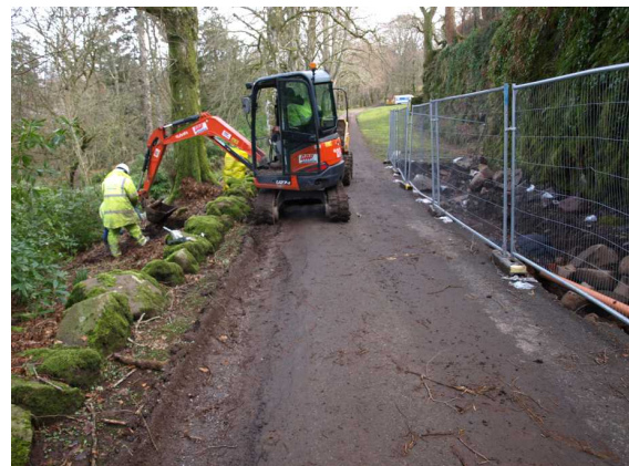
Illus 12 Clearing around outfall on N side of drive.
