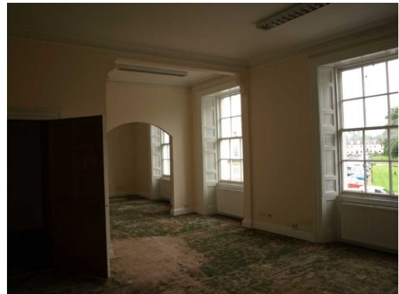
Illustration 19: First Floor, N Rooms. Moulded plaster cornice and corbels. Arched partition leads to NW room.
