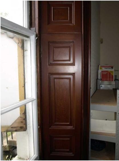
Illustration 16: Ground Floor, NW Room. Shutter with oak woodgrain effect.
