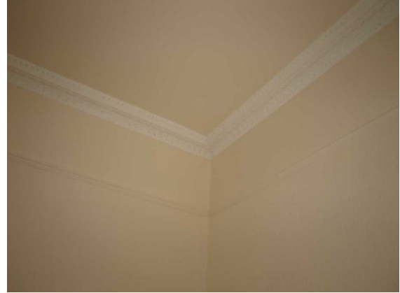
Illustration 14: Ground Floor, NE Room. Moulded plaster cornice.
