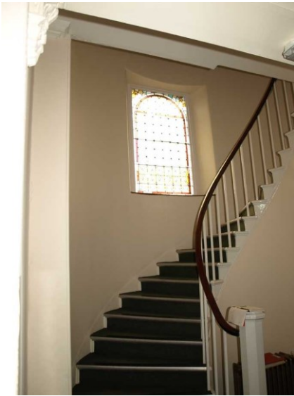
Illustration 17: Spiral stair. Cantilever stone treads. Wrought iron banister with mahogany handrail. Stained glass window.
