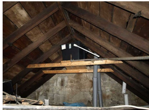
Illustration 26: Rafters, sarking boards and E party wall.
