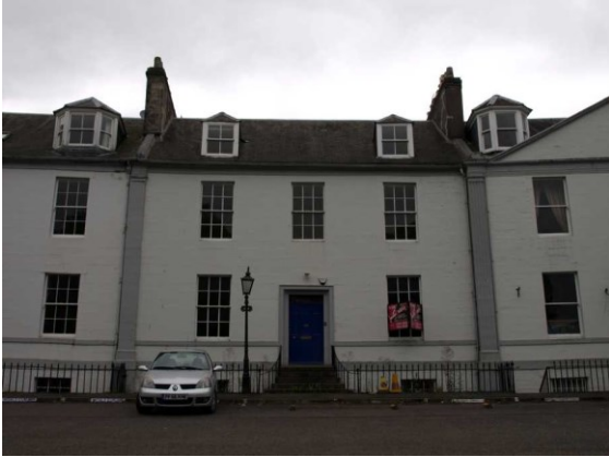
Illustration 11: Atholl Crescent facade. Lamp post to L of entrance.
