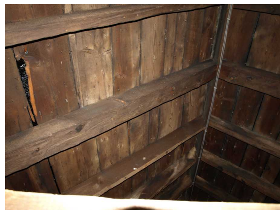
Illustration 25: Rafters and sarking boards. Double thickness rafter overhead, with interrupted ridge beam.
