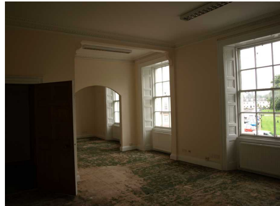
Illustration 19: First Floor, N Rooms. Moulded plaster cornice and corbels. Arched partition leads to NW room.
