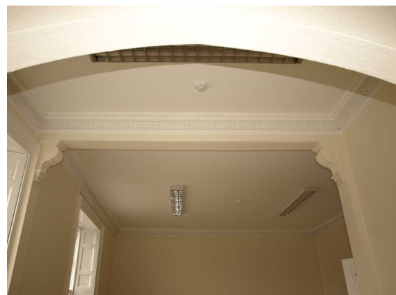
Illustration 20: Central bay, with moulded plaster cornice and corbels. Arched partition overhead.
