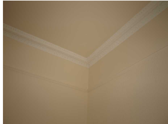
Illustration 14: Ground Floor, NE Room. Moulded plaster cornice.
