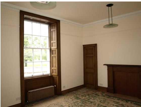
Illustration 12: Ground Floor, NE Room. Window shutters. Oak finish fire surround. Moulded plaster cornice.
