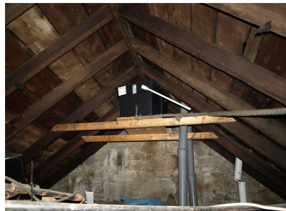
Illustration 26: Rafters, sarking boards and E party wall.
