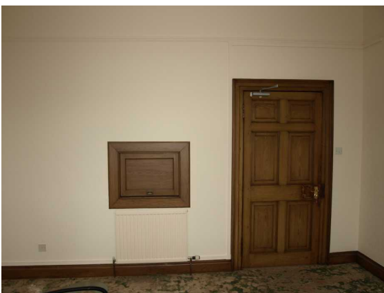
Illustration 13: Ground Floor, NE Room. Serving hatch and wide door.
