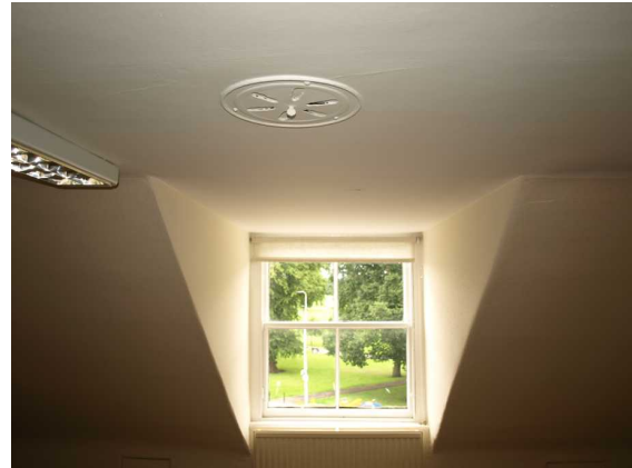
Illustration 24: NE dormer. View to North Inch. Vent overhead.
