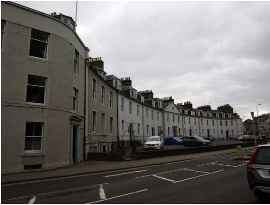
Illustration 31: Atholl Crescent with pediment at No 5. Lamp post only at No 4.
