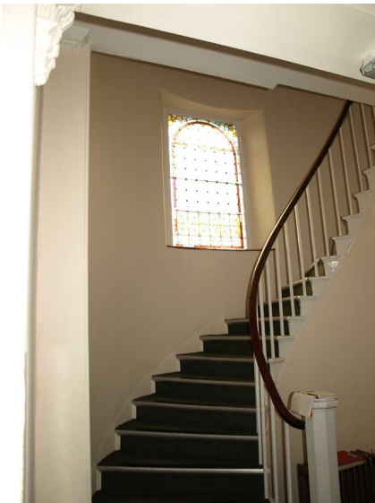
Illustration 17: Spiral stair. Cantilever stone treads. Wrought iron banister with mahogany handrail. Stained glass window.
