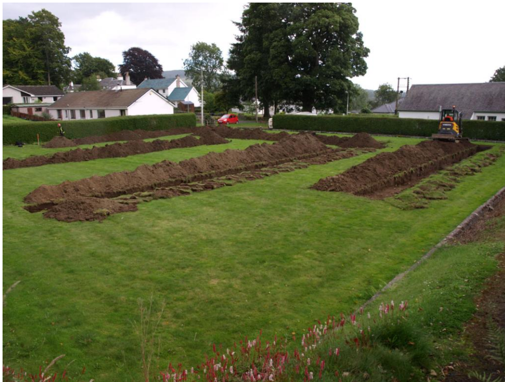
Overview of site, all trenches completed
