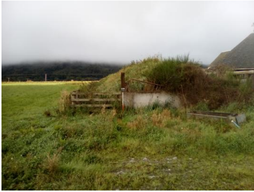
NE end of berm, banded soil from shed
