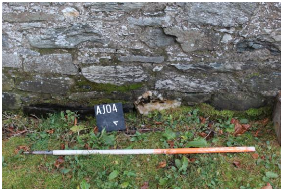
Witch stane? In exterior SW elevation of NW barn
