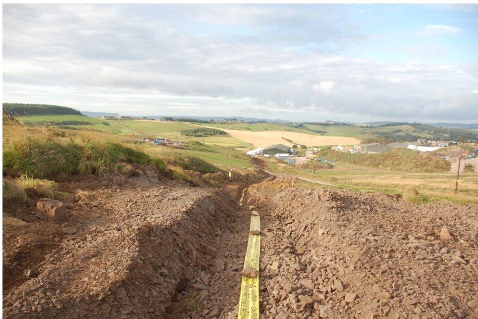
Illus 13: Narrow cable track view SW
