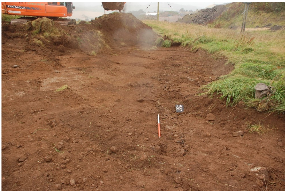
Illus 14: General stripping turbine base 04, showing field drain 0404, view SW
