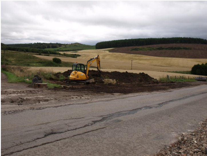
Illus 3: Forming site entrance, view SE
