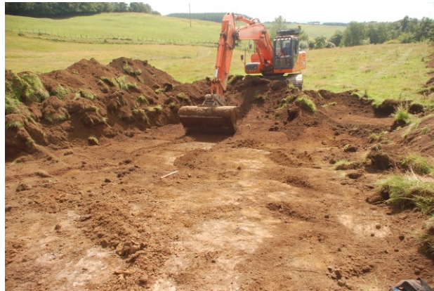
GF05: general excavation at turbine 03, for SSE compound, view SW
