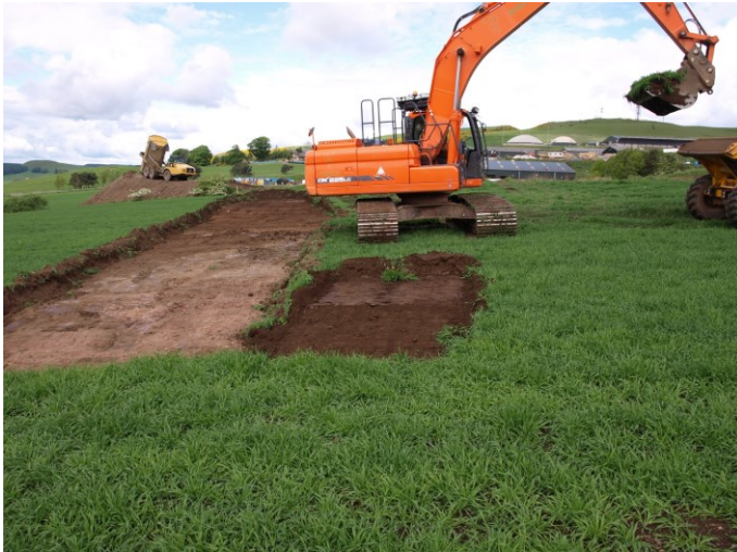
Illus 5: Stripping topsoil for turbine base 01, view NW
