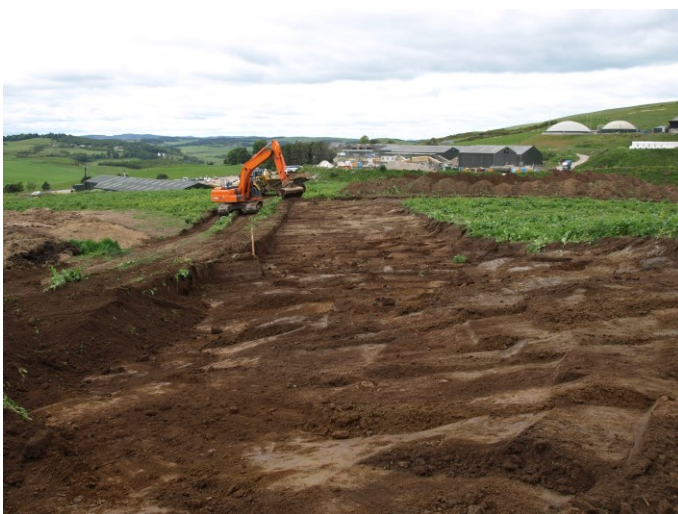
Illus 6: Turbine base 02, S end boundary strip complete, view W
