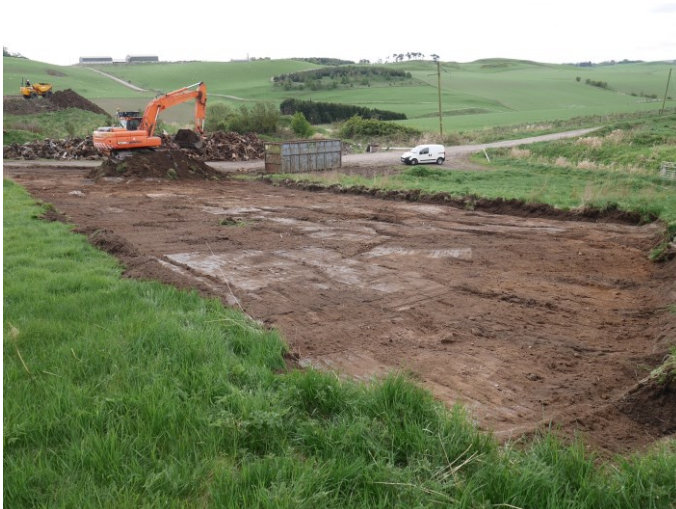
Illus 4: Forming site compound and access, view SW
