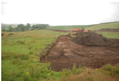
Illus 7: General stripping base 03, view W
