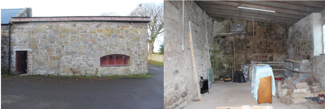
Exterior, NE elevation (workshop)
