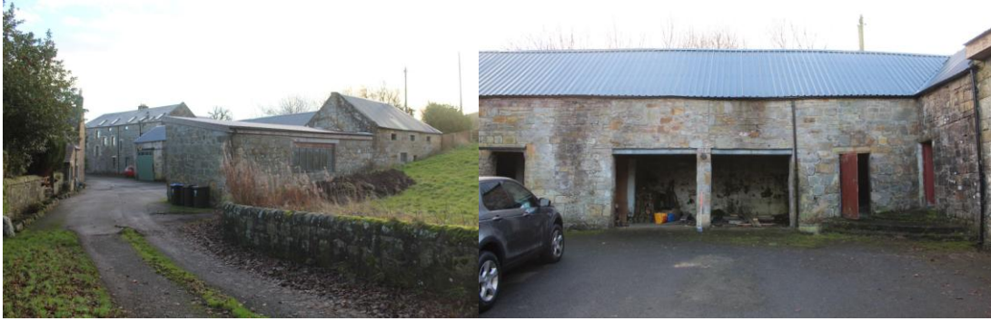
Location shot, steading with mill
