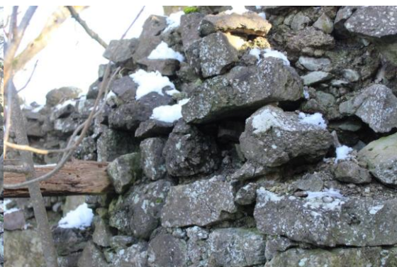
Beam slot, interior ESE elevation of cottage
