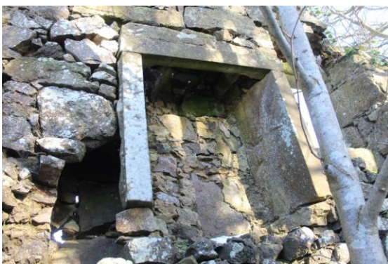
First floor fireplace, NNE elevation of cottage
