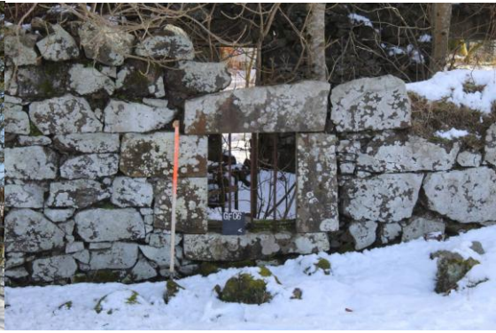
Barred window, WNW elevation
