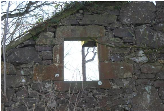
First floor window, NNE elevation
