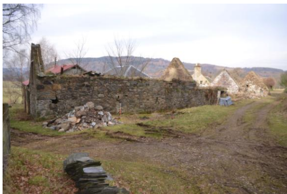
SE elevation, stone steading
