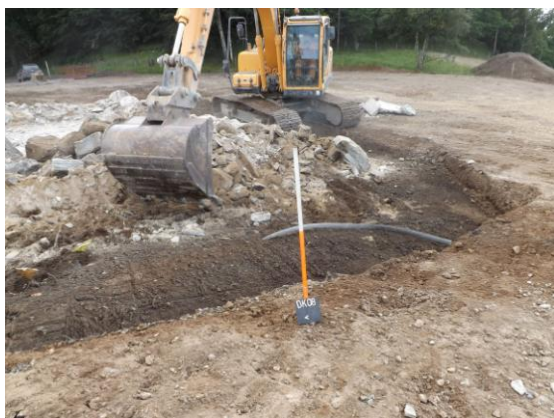
Demolition of cottage
