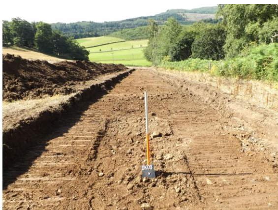
New access road, post-strip
