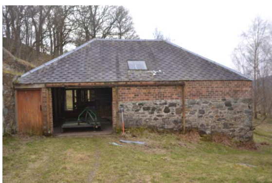
NE elevation of brick barn
