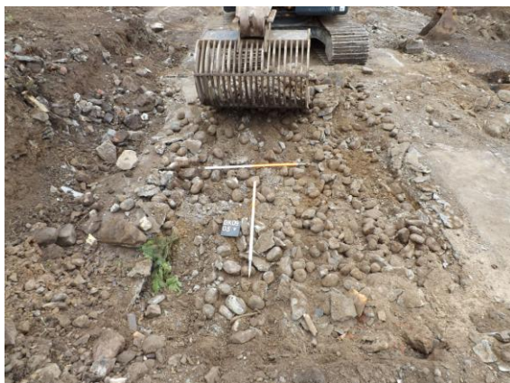
Cobbles (05), bedding for concrete floor of steading
