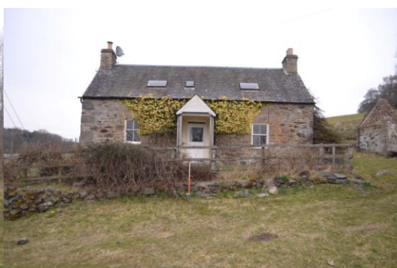
SW elevation of cottage
