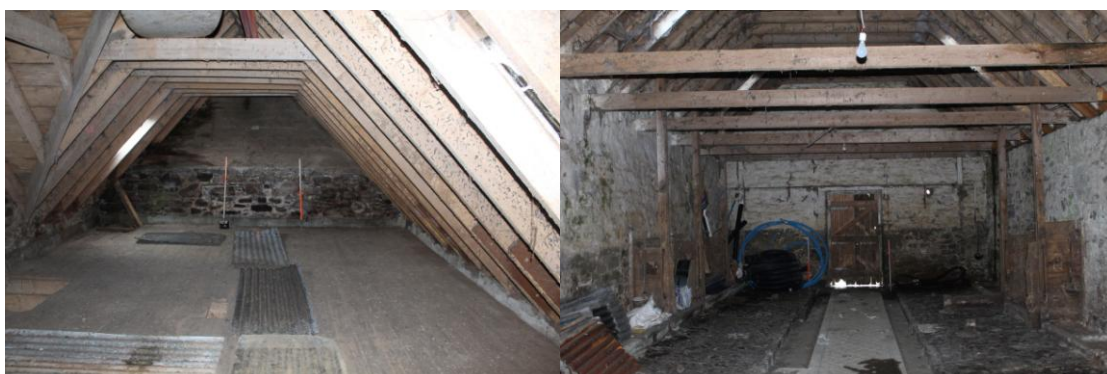
Central room, first floor
