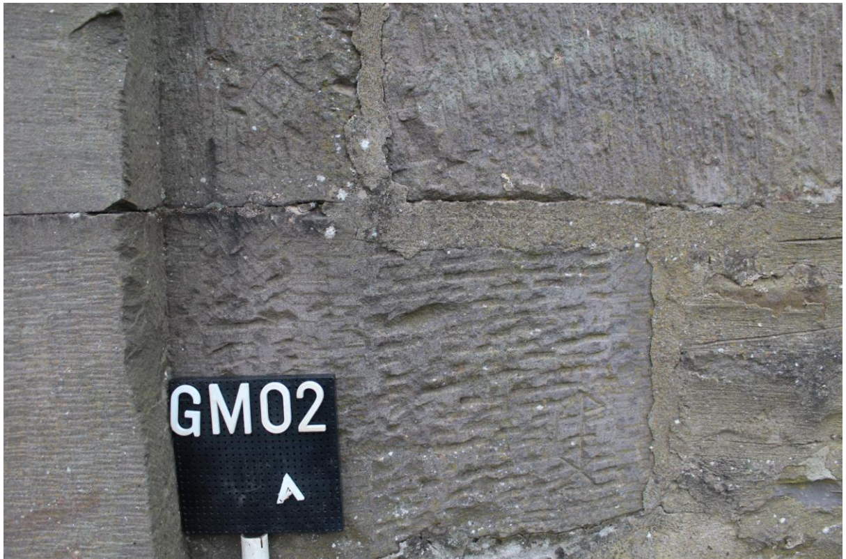
Masons' marks on S elevation of NW corner bothy (photo no. 129, see also 126-130)
