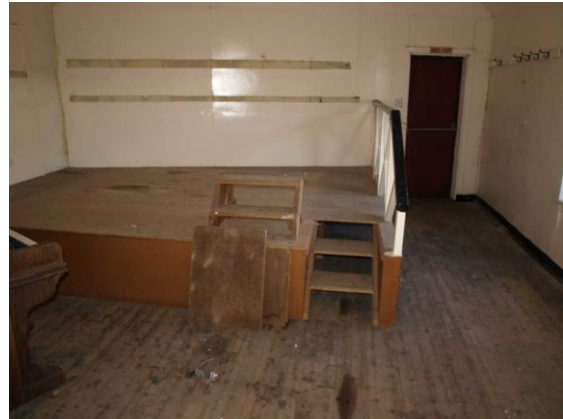
Illus 18 Upper Hall. Platform, hidden steps, and fire escape at W end
