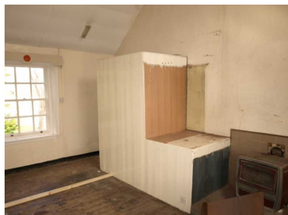
Illus 20 Upper Hall, E end. Boxed-in stair, stove. Ghost of bookshelf over stair.
