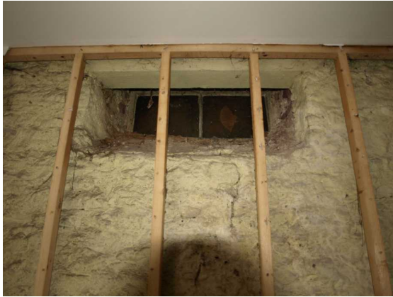
Illus 15 Blocked window in N wall
