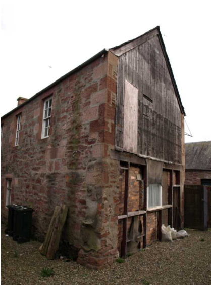
Illus 11 NW corner with rough masonry and buttress. W and N Elevations
