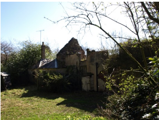
Illus 14 N Elevation and internal gable.
