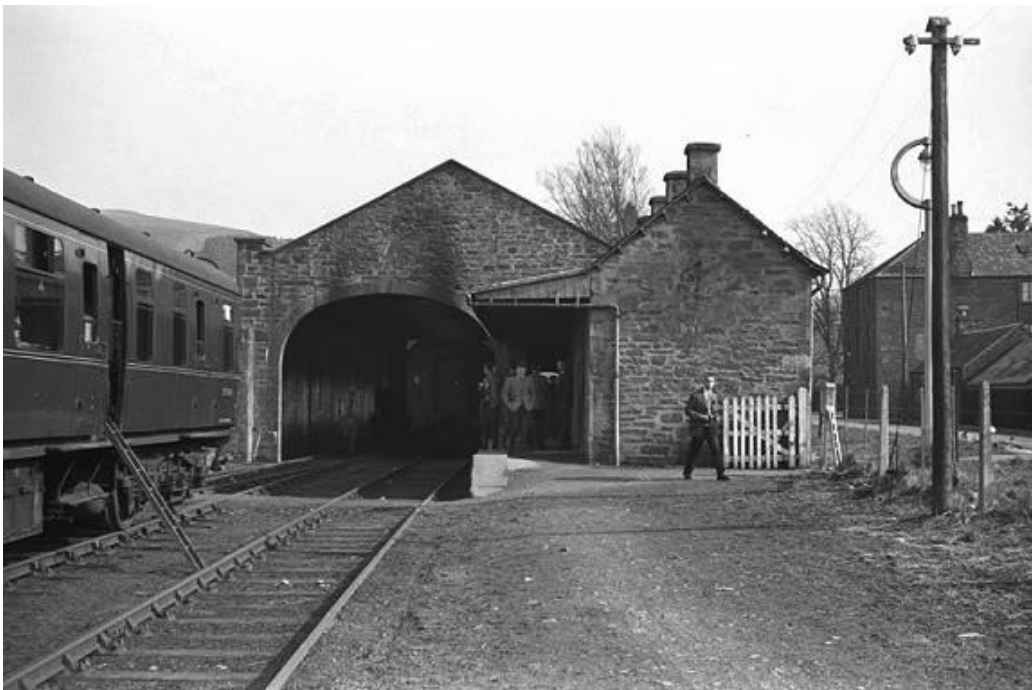
April 1962, view from N of shed, the extension shown to be a small platform with waiting rooms and veranda roof (prior to construction of neighbouring house to N on Commercial Street) (author unknown, from www.theatreorgans.com ).
