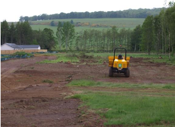
Illus 03 General work area. View N
