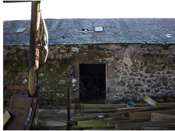
Illus 13 W Elevation. Store room door. Repointing, and change of build above lintel.
