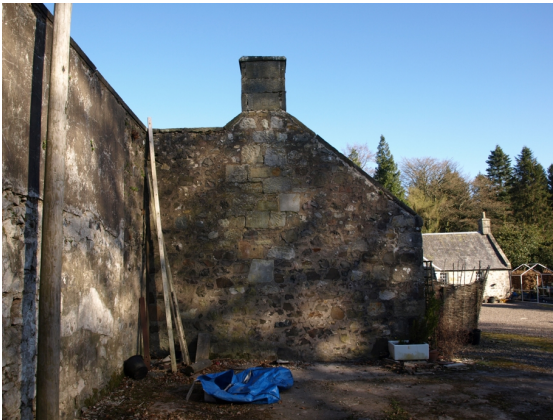
Illus 6 S gable wall.
