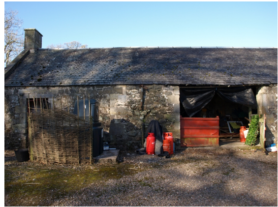
Illus 8 E elevation. Quoins show addition of S end.
