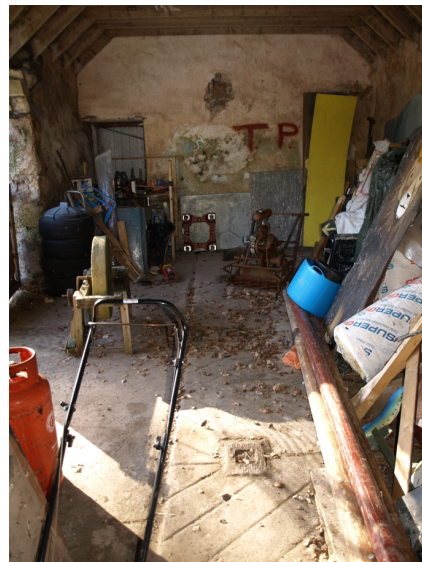
Illus 9 Stable interior. Beam end in wall aligns with post sockets in floor.
