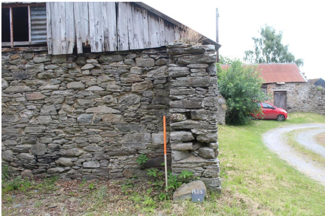
Wall stub, W elevation of E building
