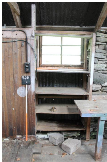
Window in blocked doorway
