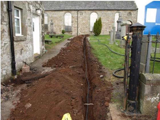
Illus 11 Trench complete, looking N
