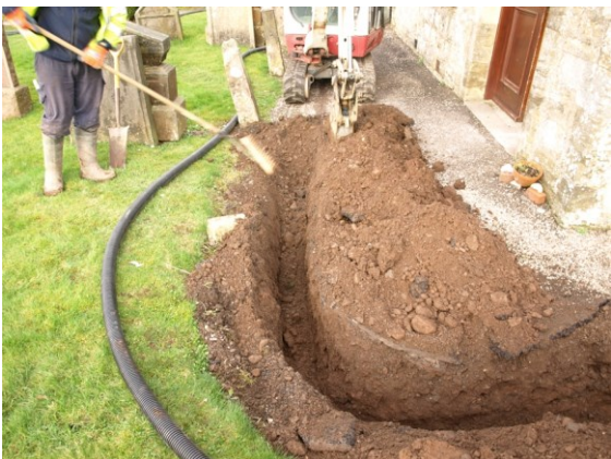
Illus 6 Trench turns W beside E door
