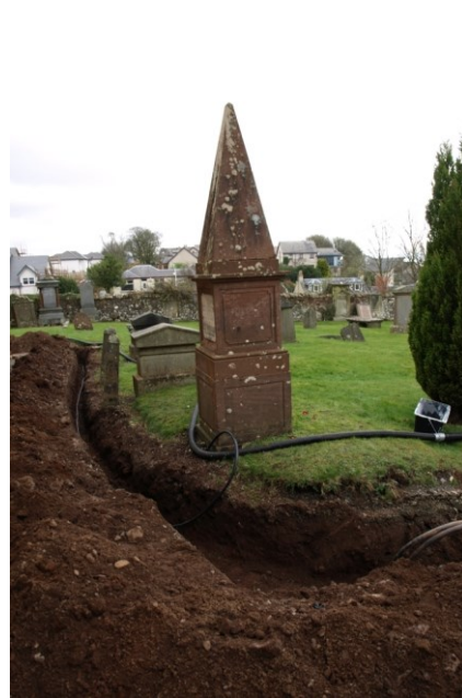
Illus 8 Trench turns S (looking E)
