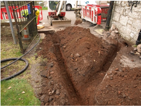
Illus 10 Trench arrives at entrance gate. Branch to cottage
