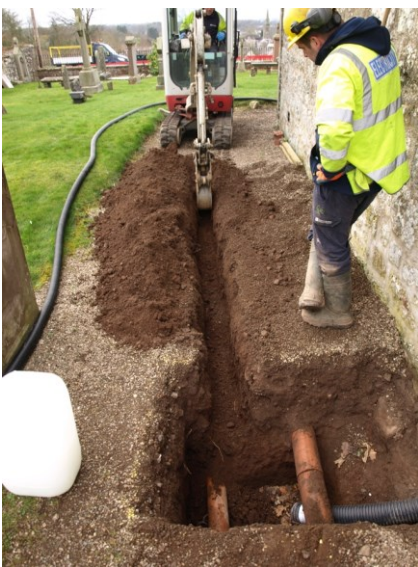
Illus 5 Initial pit beside E gable
