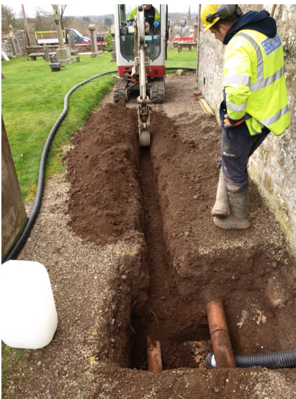
Illus 5 Initial pit beside E gable
