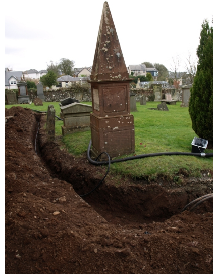
Illus 8 Trench turns S (looking E)
