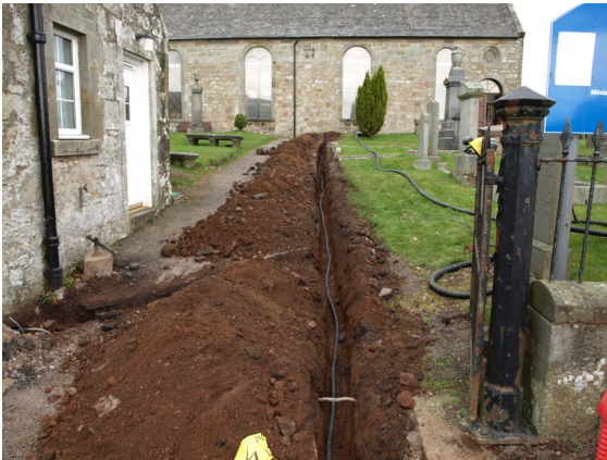
Illus 11 Trench complete, looking N
