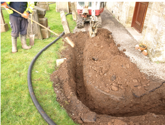
Illus 6 Trench turns W beside E door
