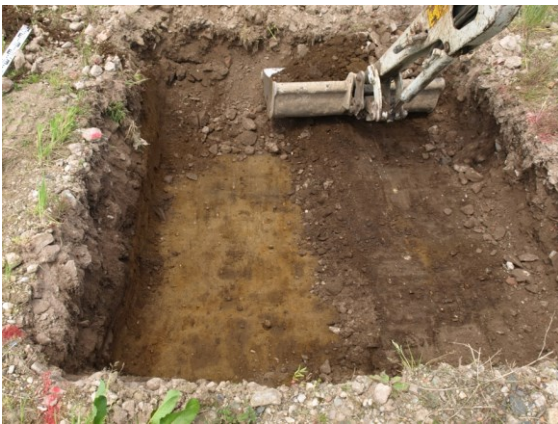
Illustration 11: Pit 09. Buried topsoil 902 over sand 903
