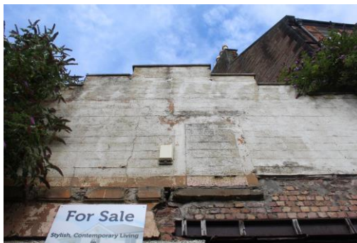
Detail, stepped gable
