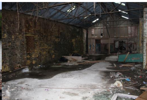
General view, interior of E building
