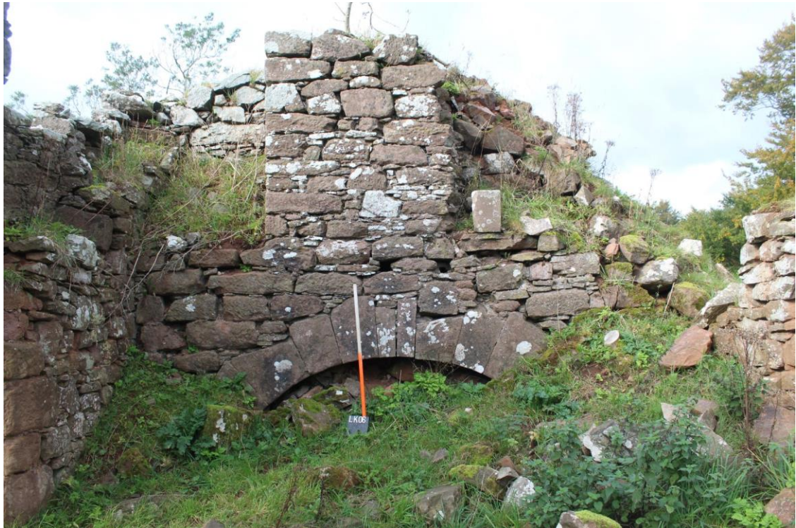
Fireplace and flue, central block main room
