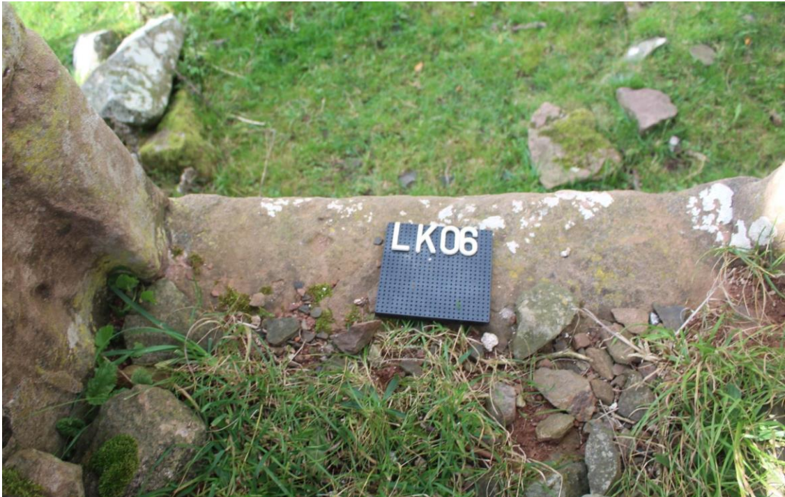
Window sill, S block
