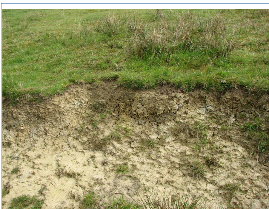
Plate 4: Exposed section of ground make-up along northern edge of Area 2
