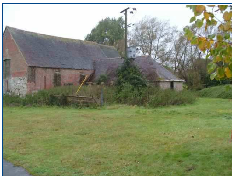
Plate 2: Area 2 looking north west
