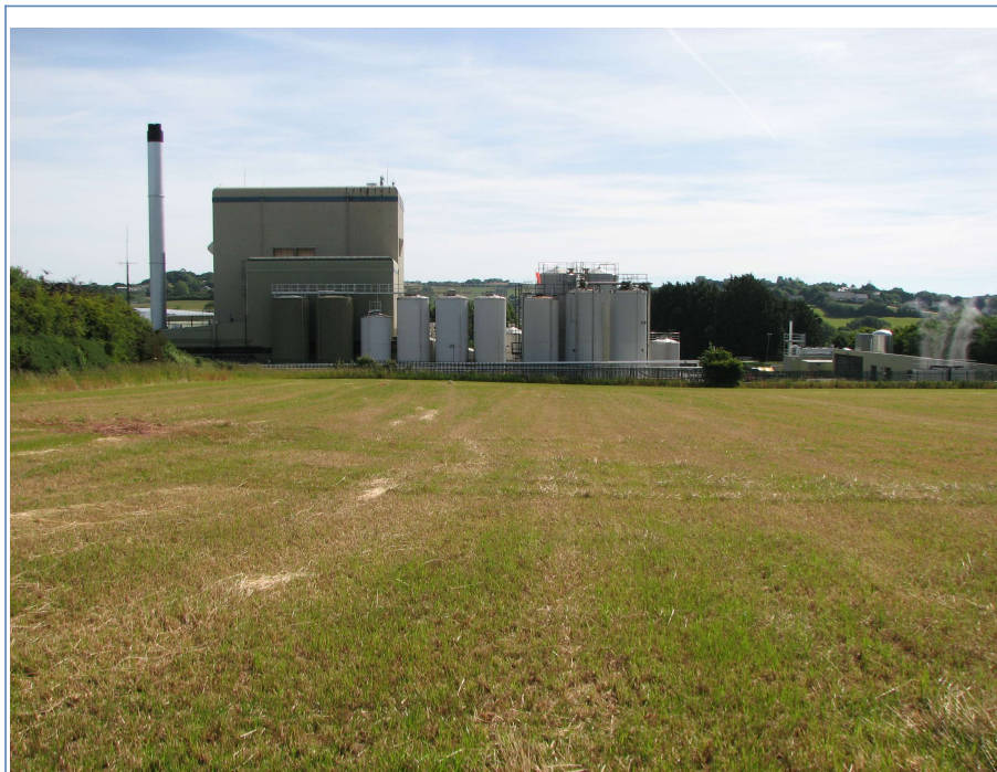
Plate 1: Proposed battery storage area looking east
