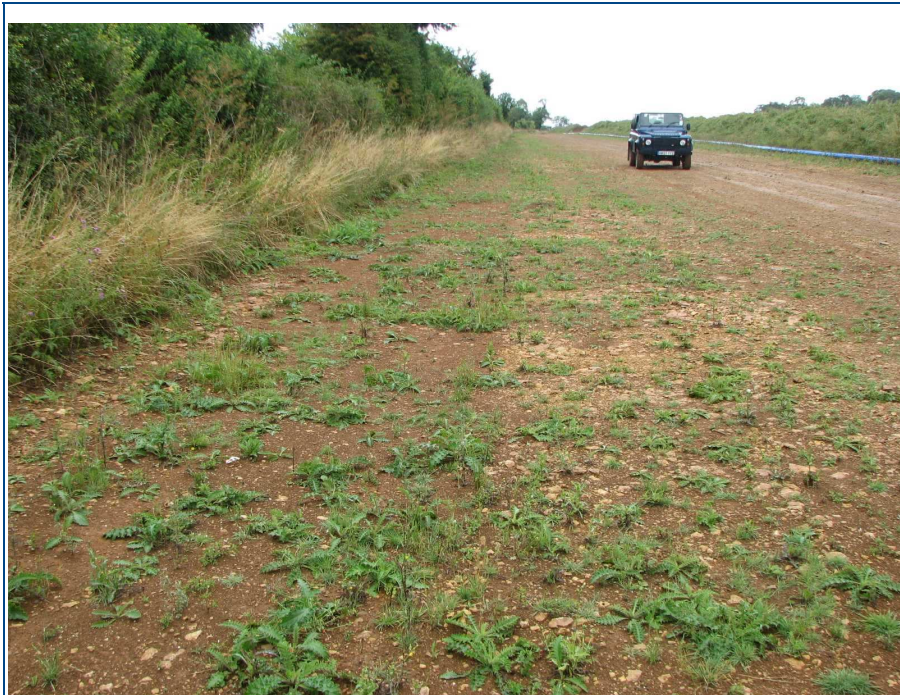
Plate 1: Area 1 - looking to the north and showing a former roadside ditch in the left of the shot
