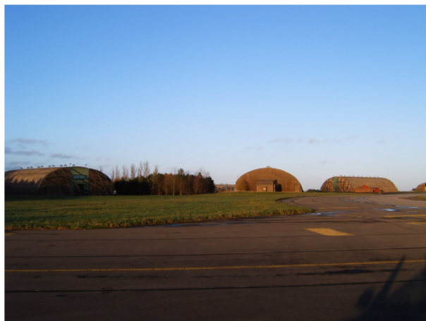
Plate 1 Central western part of survey area looking N
