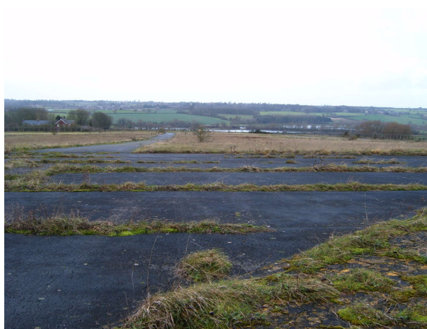
Plate 2 Western end of runway looking W
