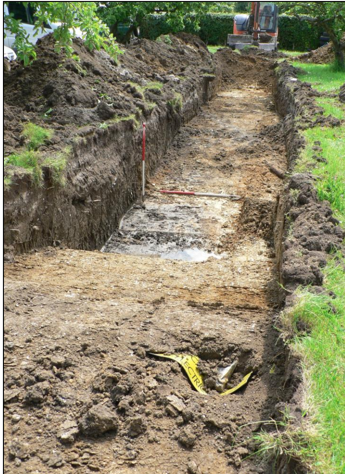
Trench from west
