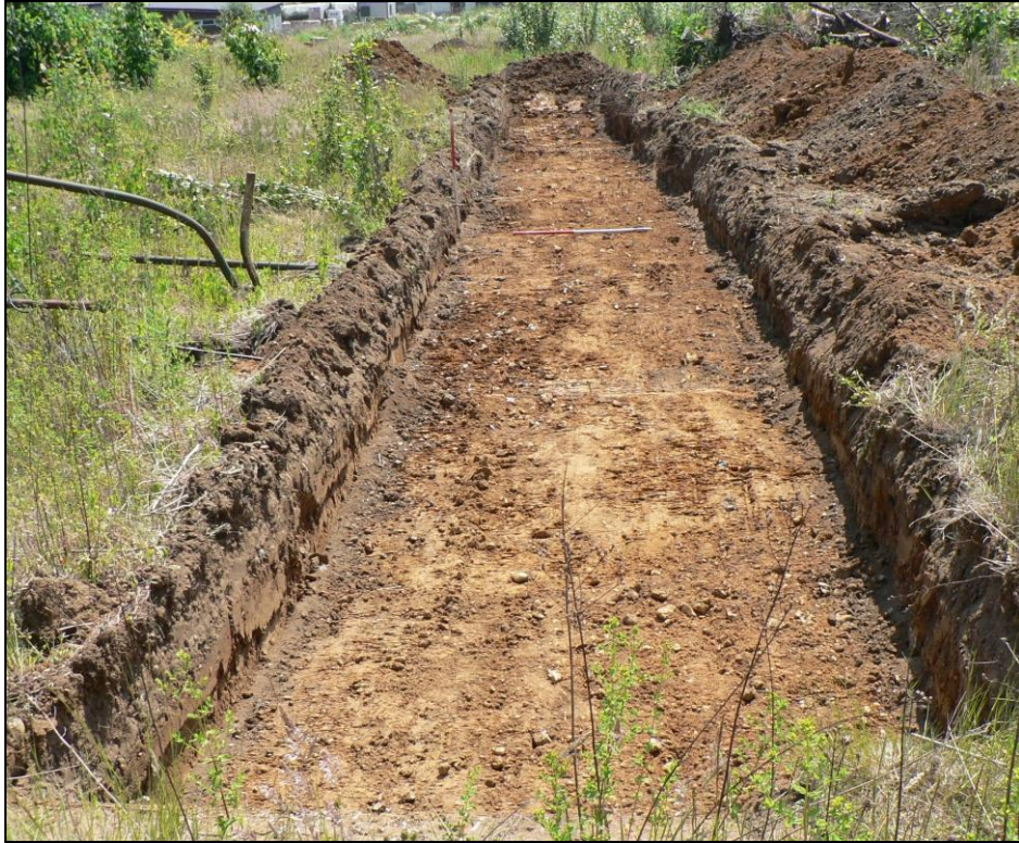
Trench 3 from northwest
