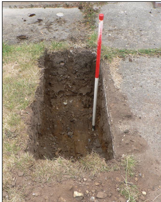
Trench for small front porch extension
