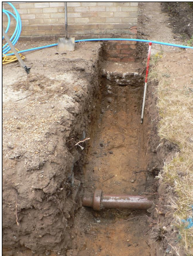
Eastern trench for rear extension
