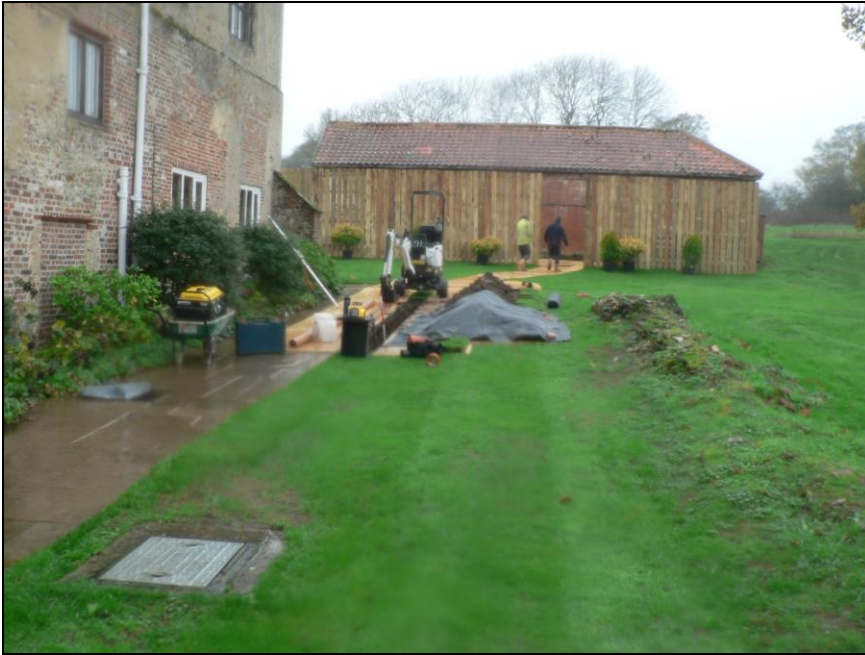
General view from east of works area with hall to left
