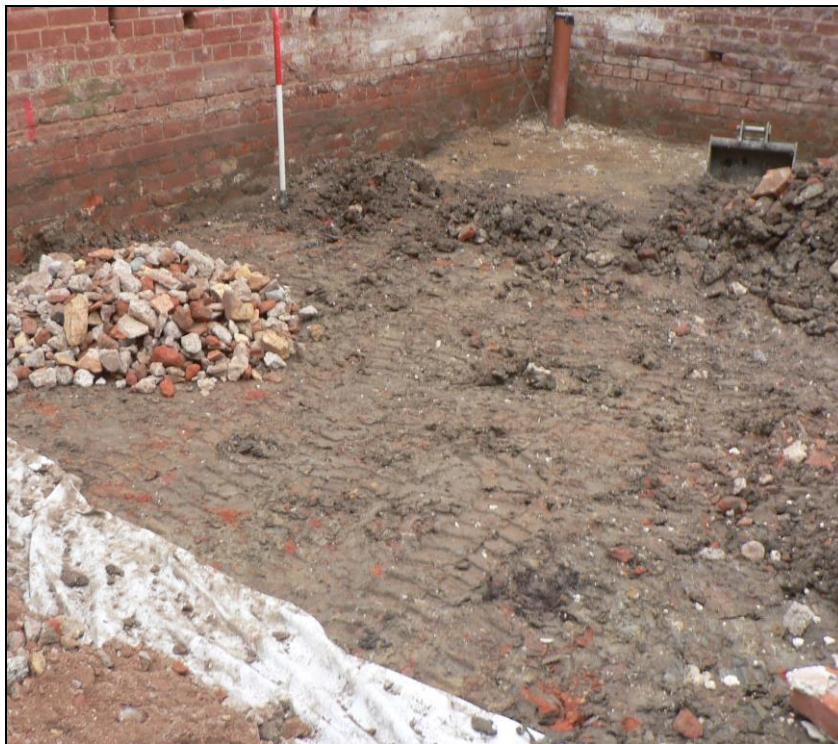
Floor lowering in eastern range of outbuildings
