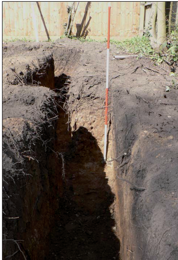
Typical trench section- eastern side of footprint
