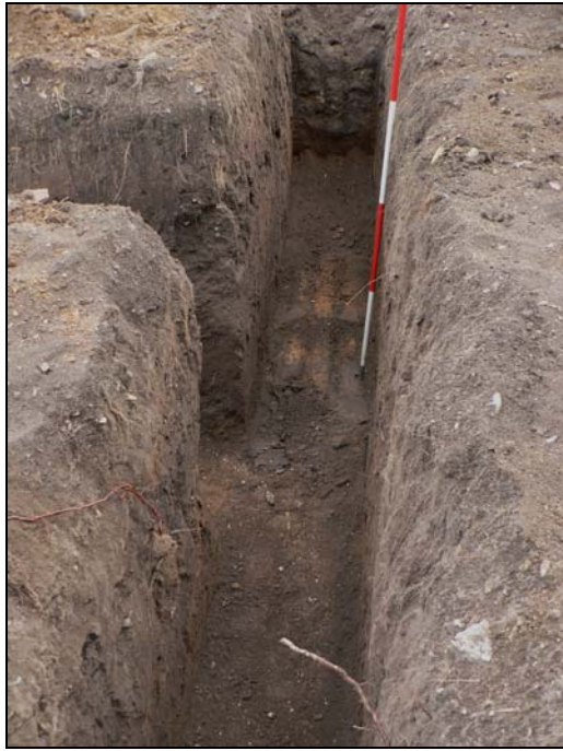
Western foundation trench from north
