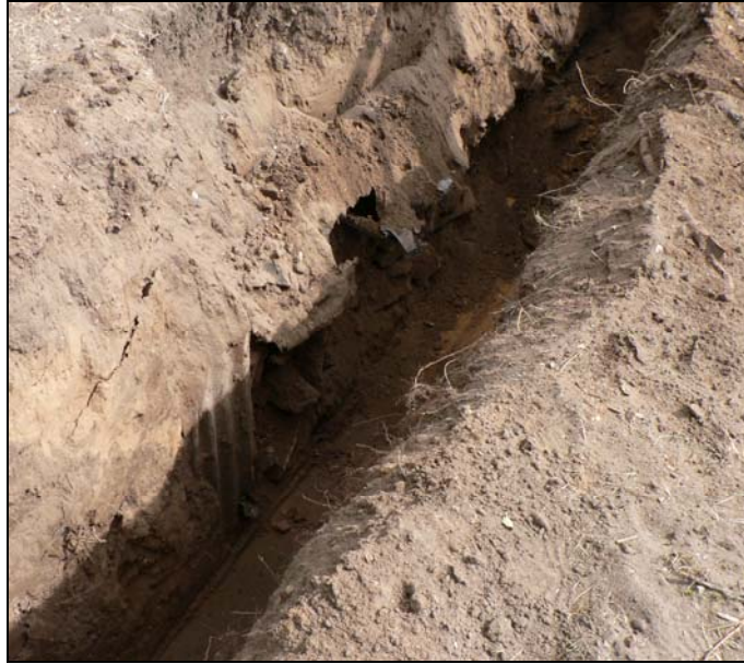
Air raid shelter in NE corner from south-west
