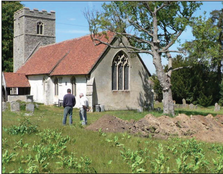
General view- T1 in foreground
