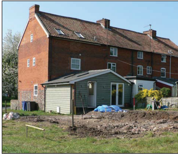
General view from north-east
