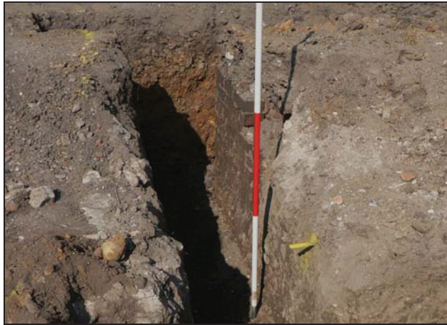
Brick foundation 0002 in background pit 0003 in foreground
