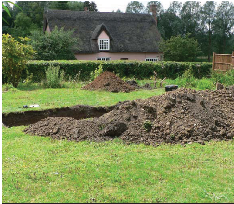
Site from north
