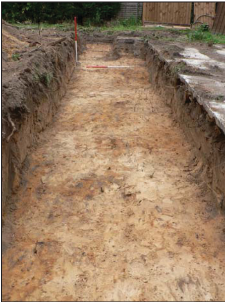
Trench from south
