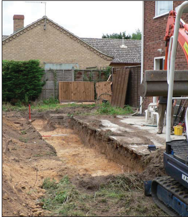
Site from south
