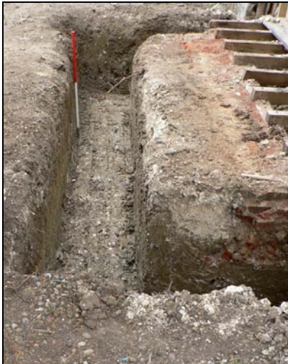
Small extension foundation from south
